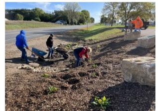
This rain garden is an example of a practical way to help increase rainwater infiltration in order to decrease its ability to cause erosion and carry pollutants. Check it out next time you are at the Town Hall!
